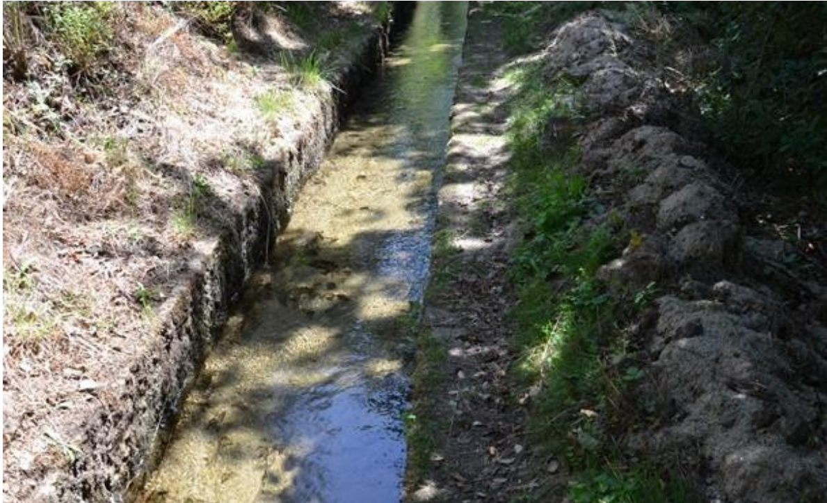
Photo 1 - Sedimentary material deposited in the channel that has its transport capacity reduced during periods of low flow.
