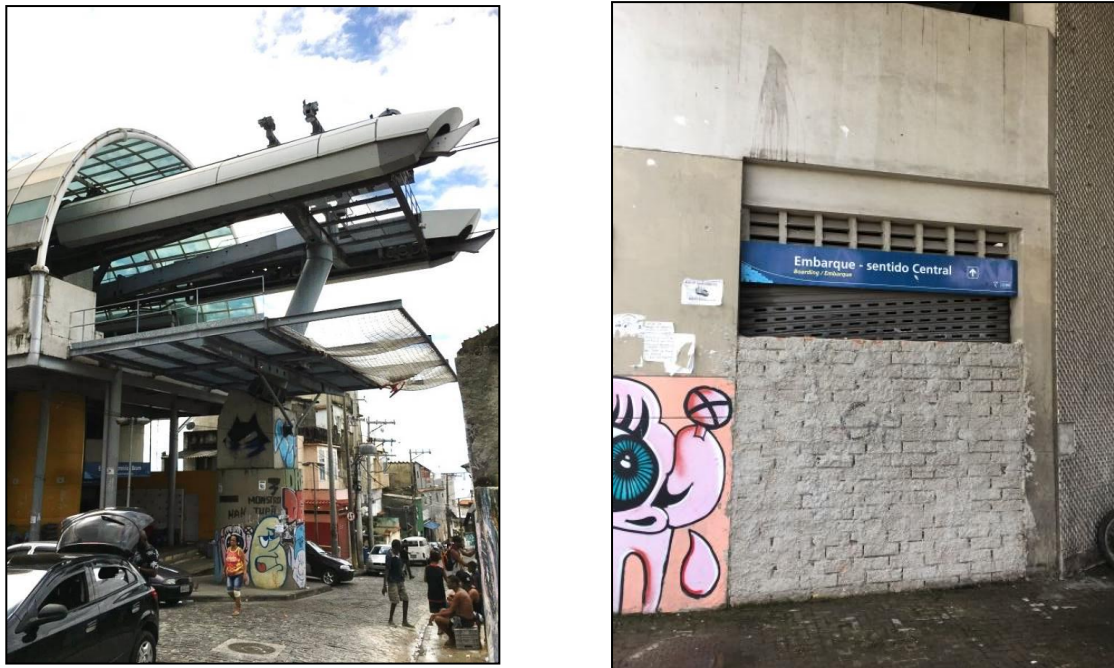
Photo 1- Providência cable car with the boarding gate blocked with bricks bricks 6
